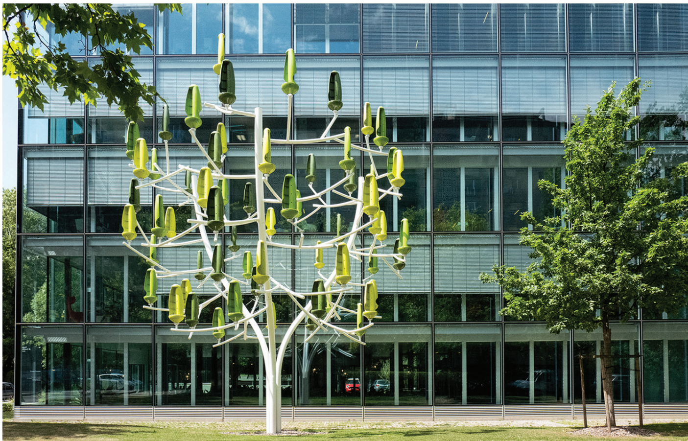
Piguet Galland & Cie SA, administrative headquarters in Geneva, Switzerland. In 2016, Piguet Galland acquired its Arbre à Vent® from the really first series of this urban wind turbine designed by world famous Swiss designer Claudio Colucci. It is a silent sustainable energy solution. It offers an average power of 3 kW and could power 25 streetlights or provides the electrical needs of a 4-person household (excluding heating).
